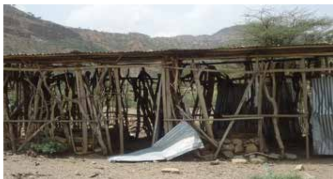
The old school structure. Photo: PCDP III/Abera ABA.
