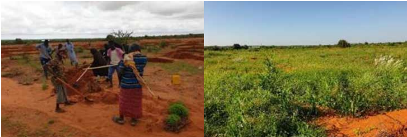
PRM before and after – community land restoration works using soil bunds, check dams and area enclosure. A photograph from Gawido Village in Beled Hawa district, Somalia. In the second picture grasses and other herbaceous types of forage plants have sprouted in the areas rehabilitated through area enclosures, soil and water conservation measures, and re-planting/reseeding. Photo: BORESHA.
