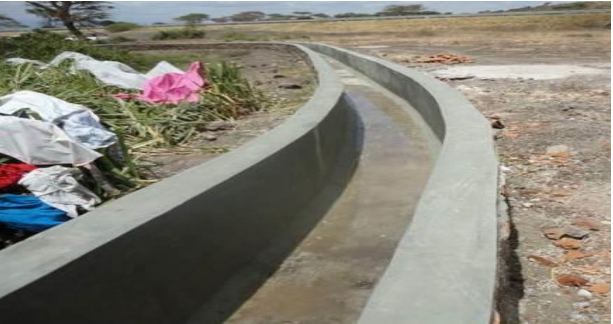
Irrigation canals at Isinet in Kajiado County
