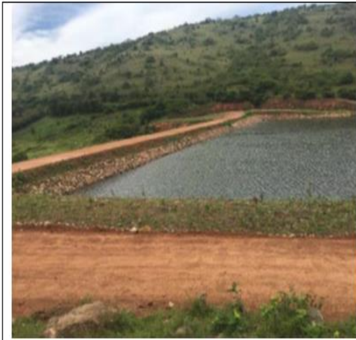
Photo 3.5.1 Status of Kagango dam in Isingiro District
