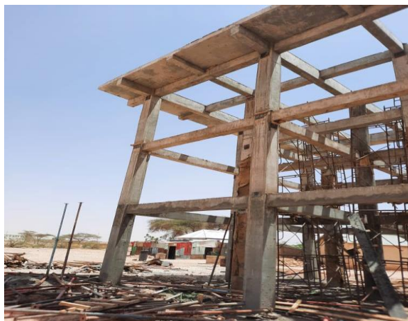
DE-SHUTERING OF THE TOP BEAMS AND SLABS OF QARDHO WATER TANK
